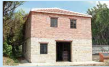
▲ Exterior of a scaled replica of the residence built in 1858 for lower-rank foreign customs officers, mostly Brits. Although modeled after English customs houses, the two-layered façade of sandstone blocks and bricks that mark the first and second stories is an innovation designed to protect against water infiltration.
