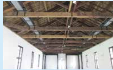
▲ Interior of the second floor of the customs official's residence modeled after English customs houses showing king-post trusses and crossbeams mounted above white stuccoed walls.
