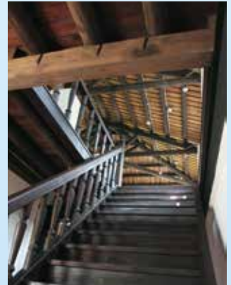
▲ Wooden plank staircase and handrail with spindle balusters leading to the second floor
