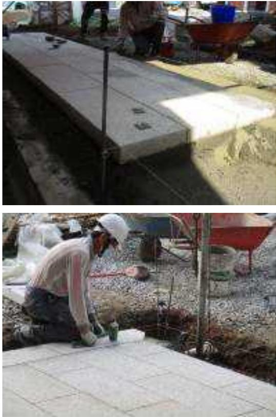
Two photographs showing the paving process. The top photo shows a worker using a long wooden stake to tap a stone slab into place. The bottom photo shows a worker kneeling and using a tool to adjust a stone slab. In the background, there is a wheelbarrow and other construction materials. |
