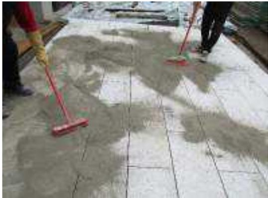
Two workers are using red-handled brooms to sweep fine sand into the joints between the stone slabs. The sand is being applied to the surface of the slabs.                                                                                                                                     |
